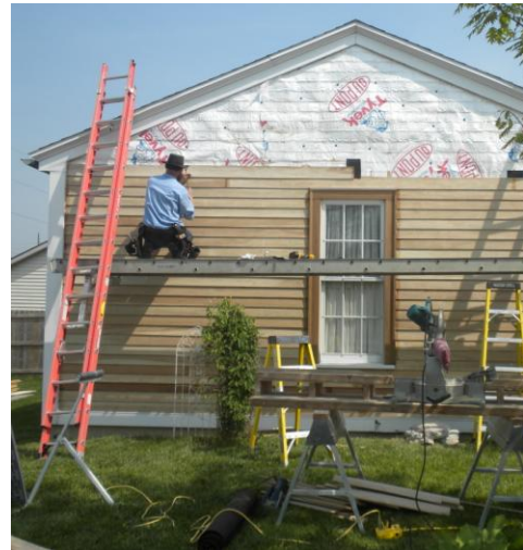
Michael O. Hunt used pressure preservative-treated yellow poplar (shown on left) to re-side his garage. His research found the wood had good paint adhesion and was resistant to fungal decay.
